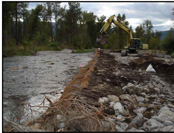
Figure B-7. Photograph showing vegetated soil lift treatment immediately after installation.
