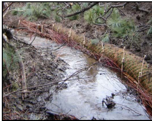
Figure B-9. Photo of installed coir log installed at the toe of a slope in conjunction with willow fascines (bottom).
