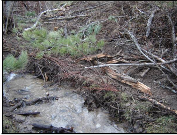
Figure B-10. Example of live willow fascines buried in the floodplain parallel to the stream. The ends of the fascines hang over the newly constructed bank.
